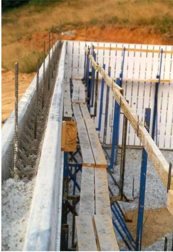
Figure 1 Sandwich Wall under Construction
